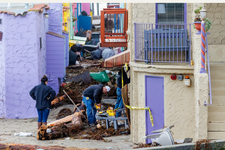
Damage to Capitola Village on Jan 5 / Kevin Painchaud
